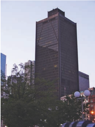
One Boston Place, third tallest building in Boston
